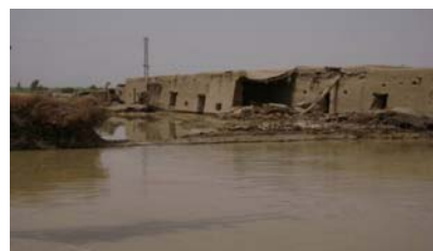
Collapsed houses at village Muradani, district Bolan
